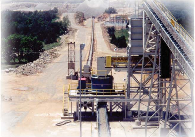
Turbo™ 175 Installation Crushing Dolomite / Limestone at 1400 TPH 24 Hours a Day / 7 Days a Week.
