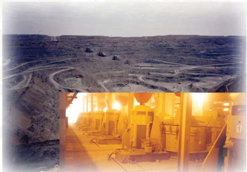
The Largest VSI Installation in the World, 16 Dual-Motor Turbo™ 96's Crushing Gold Ore at the 3rd Largest Gold Mine on Earth. This Plant Processes 1.1 Million Tons per Month.
